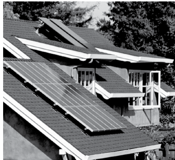
FIGURE 6-4. FLAT-PLATE COLLECTOR (BACKGROUND) AND PV ARRAY (FOREGROUND)
